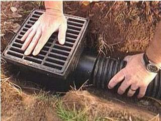
Catch basins and drain tile capture rainwater from downspouts and direct it away from foundations.
